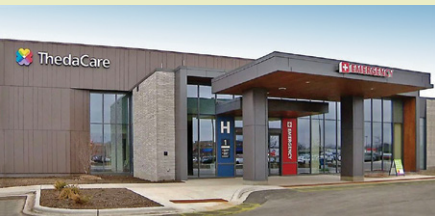
ThedaCare celebrated the completion of ThedaCare Medical Center - Fond du Lac , a new 25,000-square-foot hospital.
