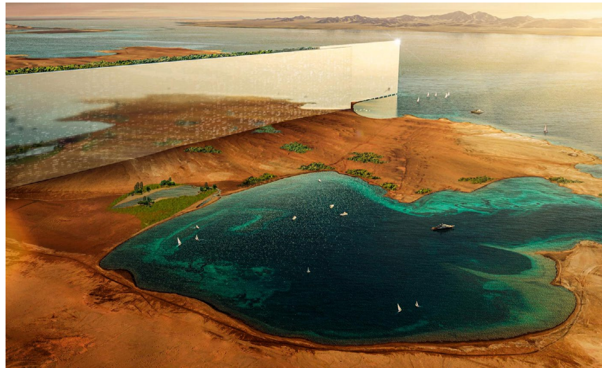
The Line, a linear smart city under construction in Neom, Saudi Arabia.
